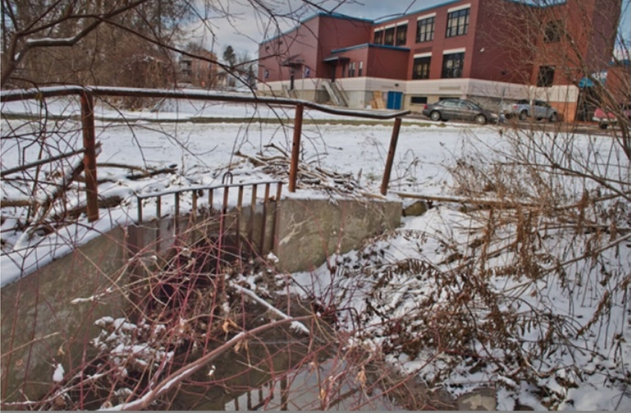
One of two inlets to the village’s crosstown canal, pictured Thursday, is at the southern end of Potsdam High School on Leroy Street. The subterranean canal moves surface and ground water across the village to the Raquette River. Christopher Lenney/Watertown Daily Times
