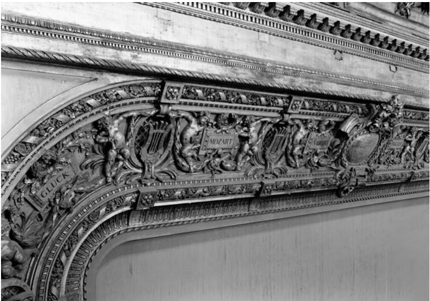
Figure 7b. Detail, proscenium arch, upper left corner, Metropolitan Opera House, ca. 1966, prior to demolition. Jack E. Boucher, Prints and Photographs Division, Library of Congress, HABS NY,31-NEYO,79-13.
